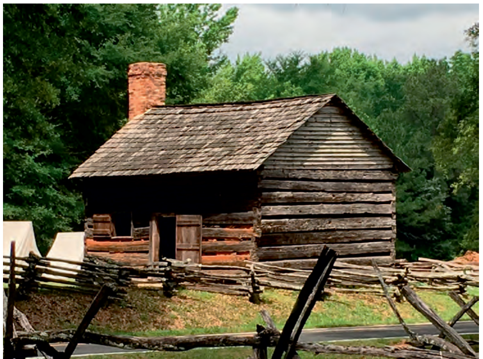
Figure 7: The slave quarters discovered by the survey may have been similar to this structure at Historic Brattonville, with the exception of a wood / clay chimney. (Photo by Chris Gillam)
