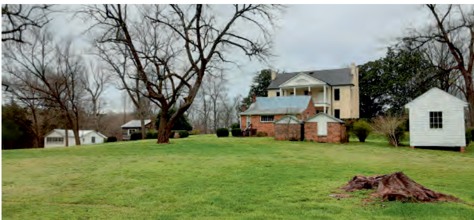
Figure 2: View of Gist mansion, kitchen, and outbuildings. (Photo by SCIAA-ARD)
